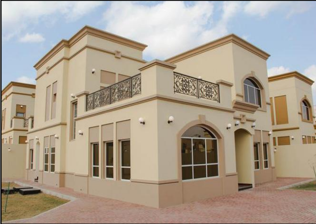
FUJAIRAH HOUSING COMPLEX
